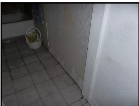
drywall damage
