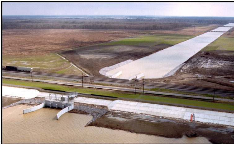
Flood control structure at Davis Pond located east of Luling, LA
