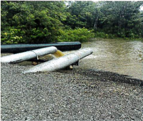
One of four pipes pumping out water Pump shut off 2 hrs after rain event
