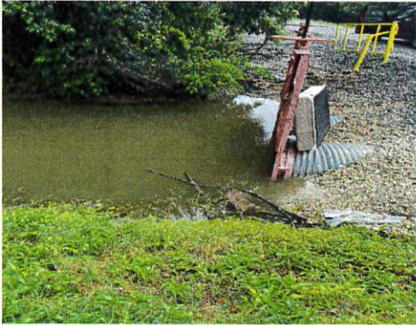
Culvert Other side of Drive to Pump Station
