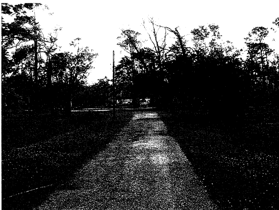
View of the existing driveway – looking east
