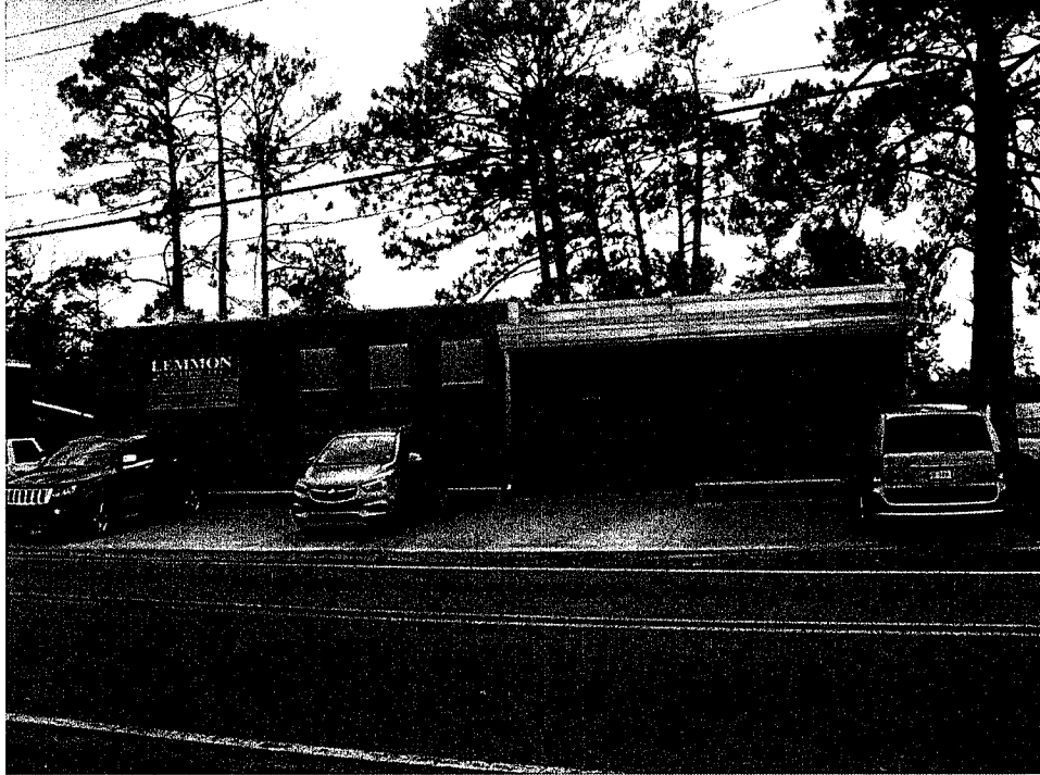
Front view of 15058 River Road from River Road - looking east
