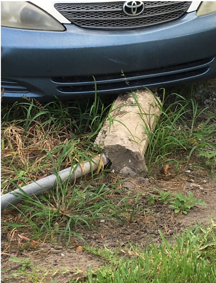
This is one of the posts of the destroyed AT&T fence with the cement that was in the ground.
