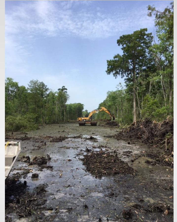
A 100' wide section of the WSLP levee footprint was cleared for surveying activities
