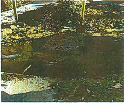
Exploratory Excavation @ Sta. 121+00. Existing D.I. discovered
