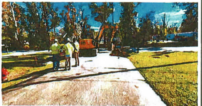
Exploratory Excavation @ Sta. 121+00. 450 Barber Rd.
