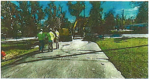
Exploratory Excavation @ Sta. 121+00. 450 Barber Rd.
