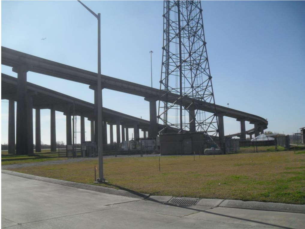
View of the subject from Deputy Jeff G. Watson Drive - looking southeast
