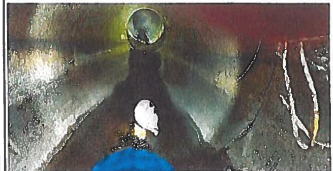
Exploratory Excavation @ Sta. 121+00. Existing DL looking from outfall at the Canal side.
