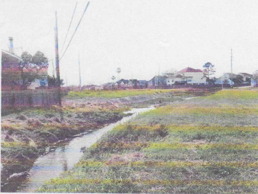
Figure 7. View looking south of culvert discharge point to Stanton Hall Canal.
