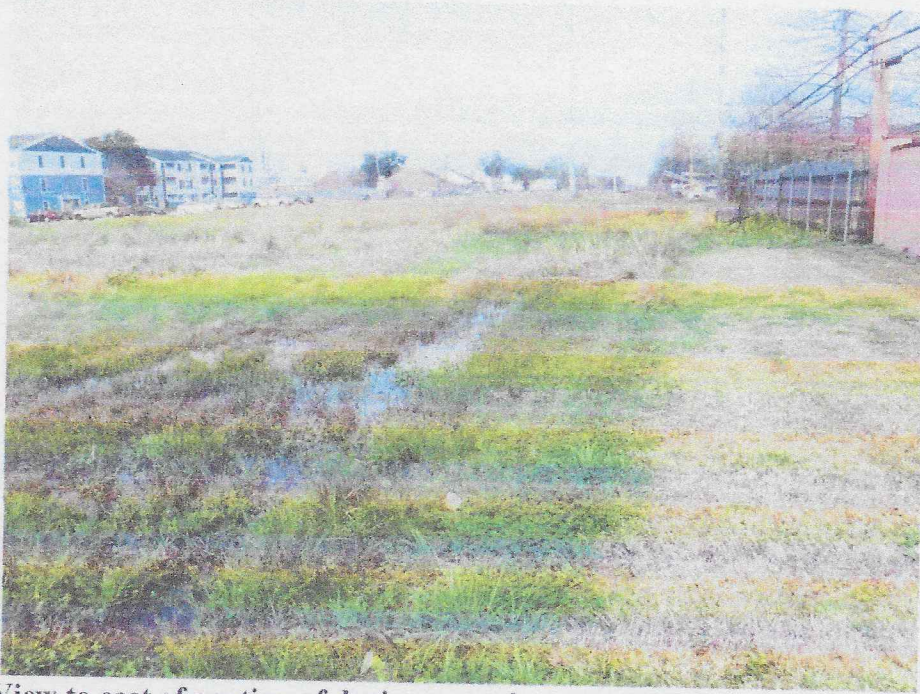
Figure 5. View to east of portion of drainage swale not yet silted up. The swale needs to be re-excavated from Ormond Boulevard to this juncture.
