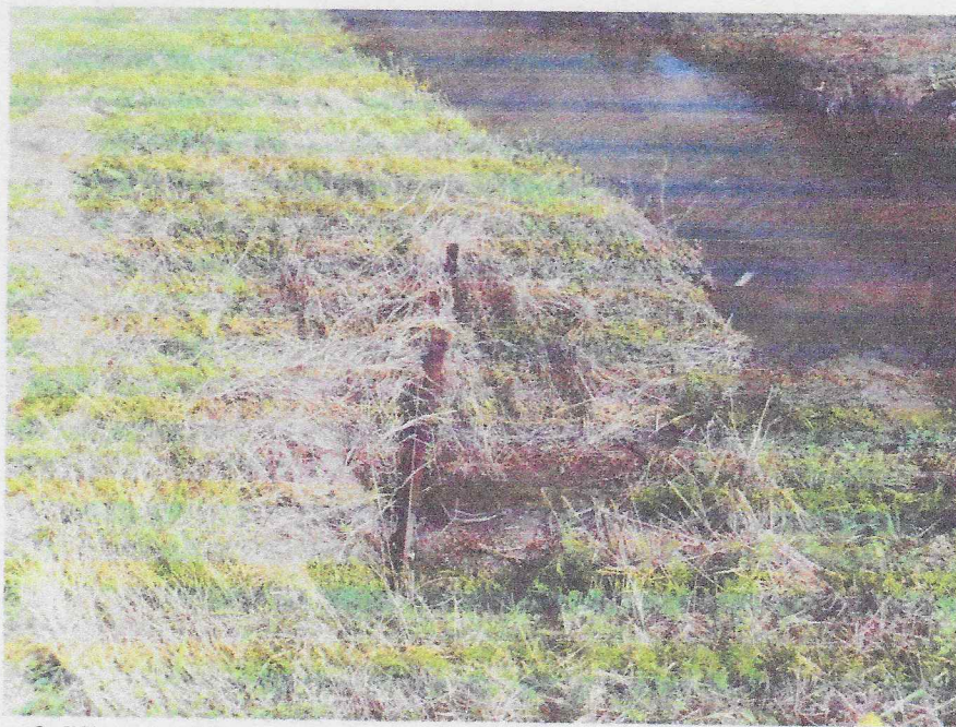
Figure 8. View looking east of culvert discharge point to Stanton Hall Canal.
