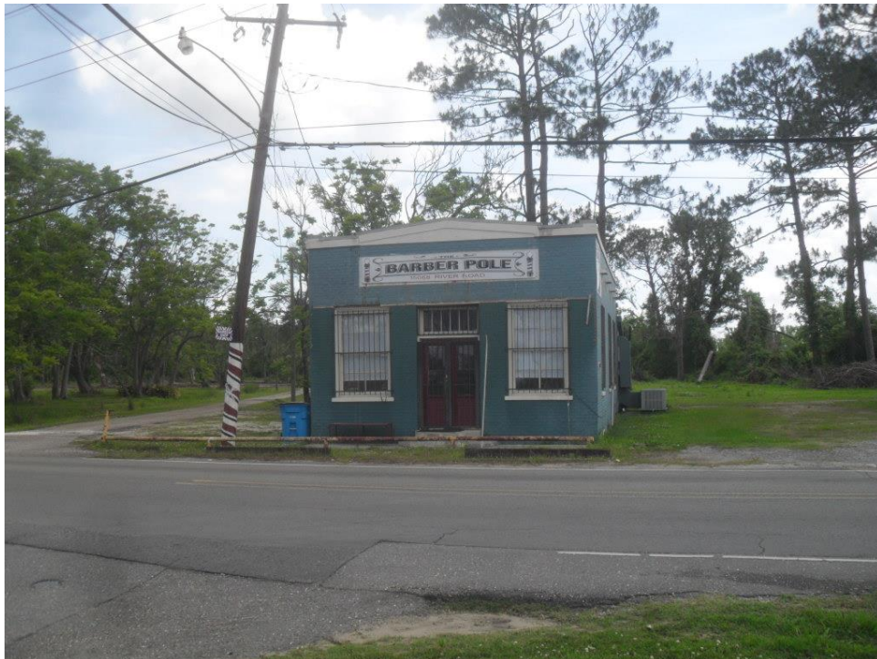
Front view of 15068 River Road from River Road - looking east
