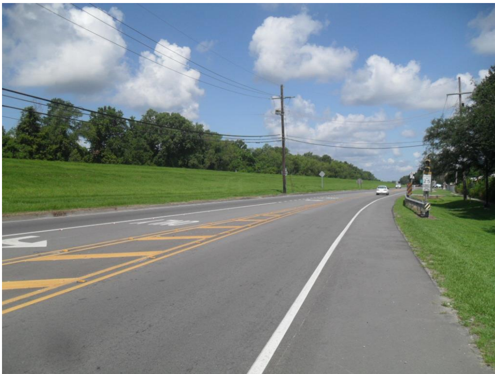
Street scene of River Road – looking west
