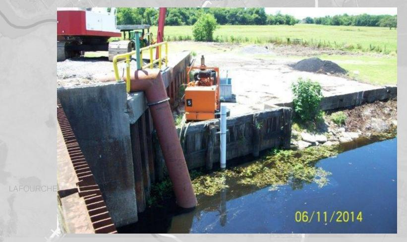
• Installed a temporary 24" hydraulic pump to offset some of the capacity lost while completing engine and pump maintenance.
