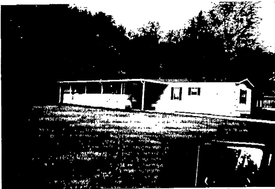
Suitable mobile home that is one of many in the area that is following zoning requirements and property is well maintained.
