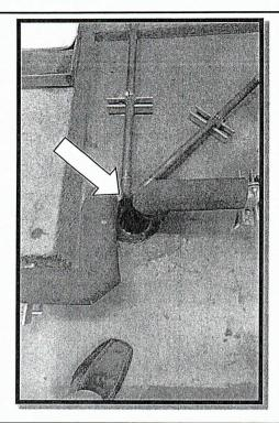
Repair conduit serving emergency pan float switch for AHU-2. Relocate float switch as necessary to avoid stepping on conduit. \$250.00
