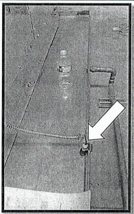
Repair chiller/boiler room floor coating. It appears that floor was damaged by welding activities during construction. \$2,500.00 Repair chiller room floor coating. It appears that floor was damaged by welding activities during construction. Patch wall opening below new Panel LC2 location. \$200.00
