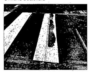
• Crosswalk striping is flaking up southbound near the railroad (2 Stripes, one on each side, intersection of Thomas Kolby)
