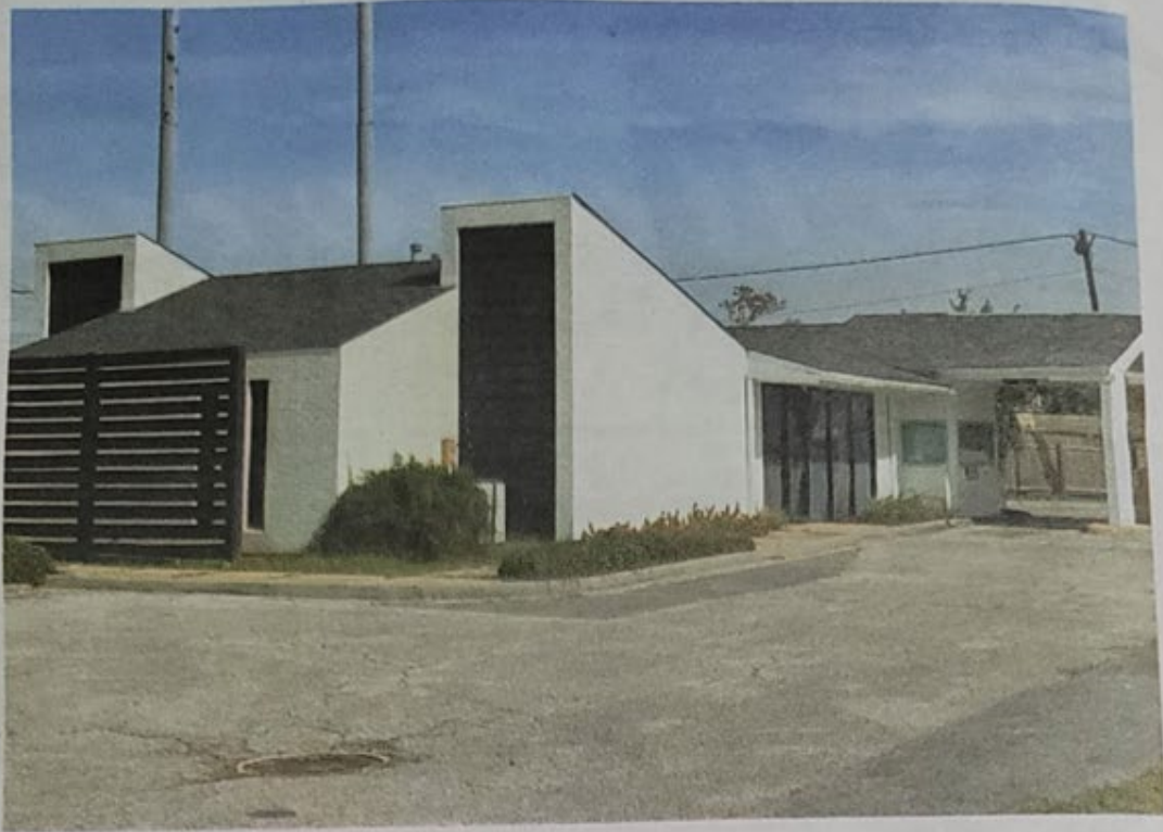
The Louisiana Business Center's Highway 90 location in Luling.
